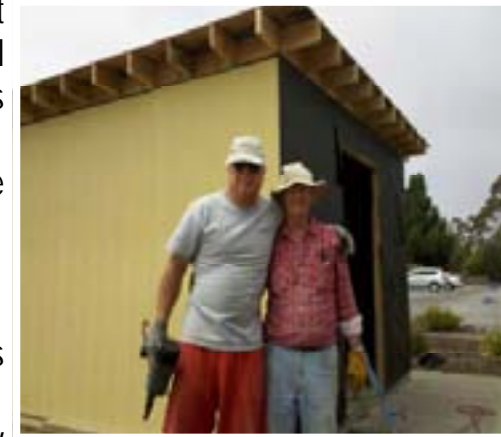
Men At Work: Norm Henderson & Tom Egan building the new shed.
