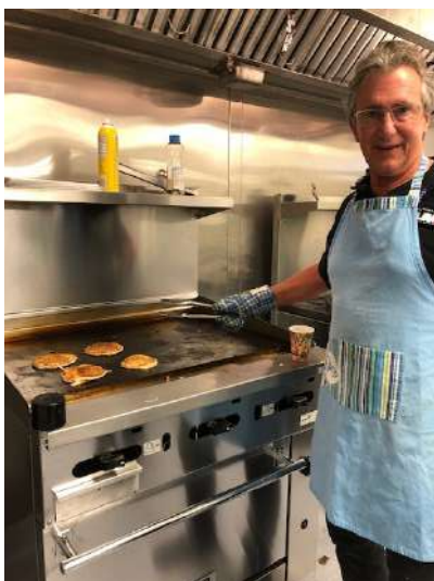
Paul making the Shrove Tuesday pancakes on the new stoves!
